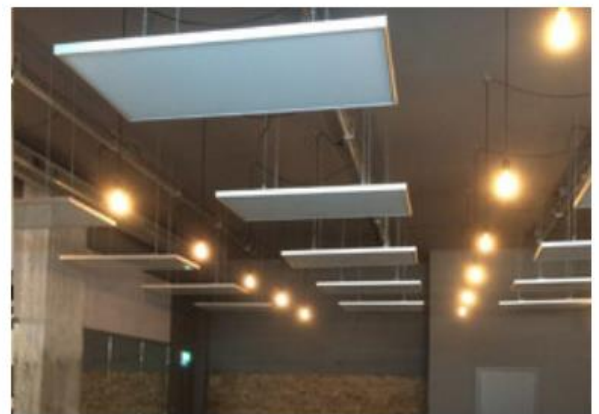
Infraroodpanelen (Bron: www.hotyogaverwarming.nl )
